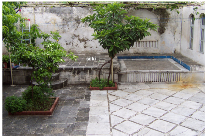
Fig.8. Specialized raised platforms ( seki ) in the courtyard, covered with grape-vine, providing outdoor dining and resting places. Antakya, 2004. (photo: author)
